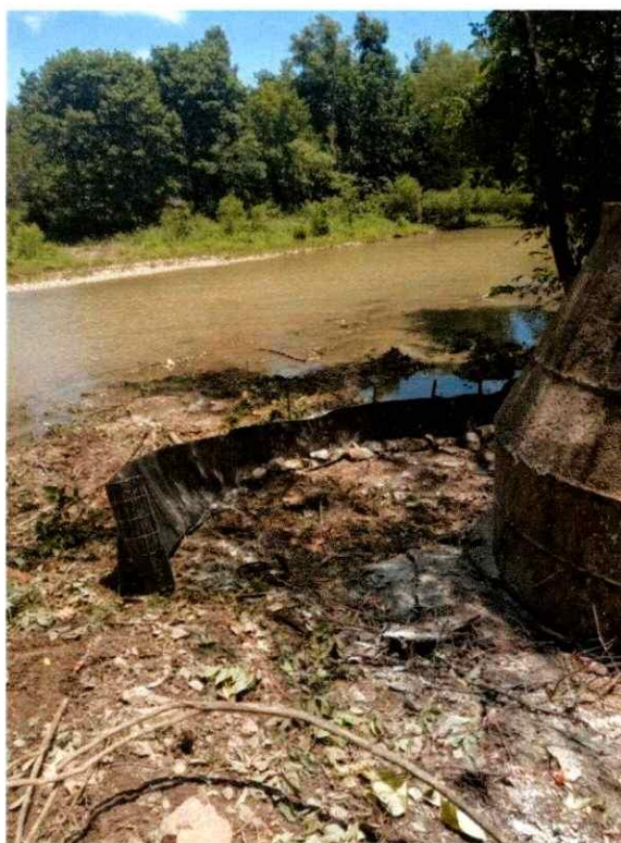
MH 1748 During Cleanup – 7/12/2024
