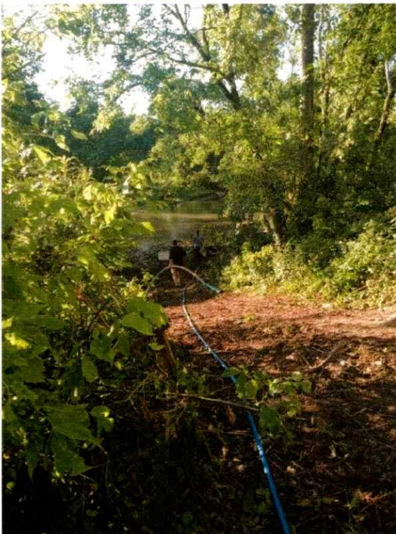
MH 1748 During Cleanup – 7/12/2024
