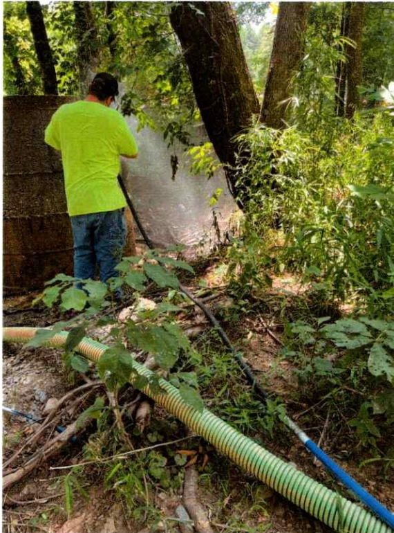
MH 1748 During Cleanup – 7/3/2024
