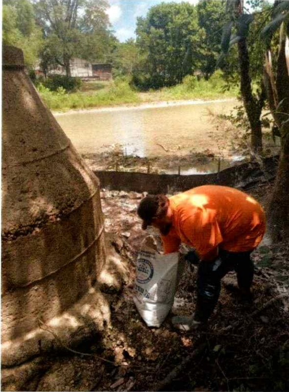
MH 1748 During Cleanup – 7/12/2024
