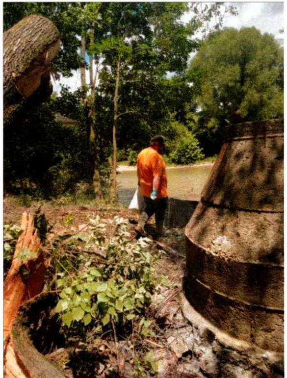
MH 1748 During Cleanup – 7/12/2024
