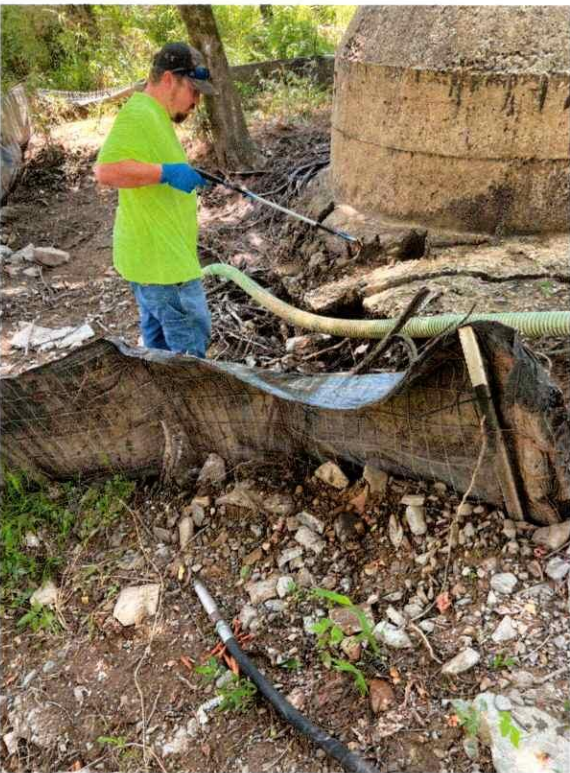
MH 1748 During Cleanup – 7/3/2024
