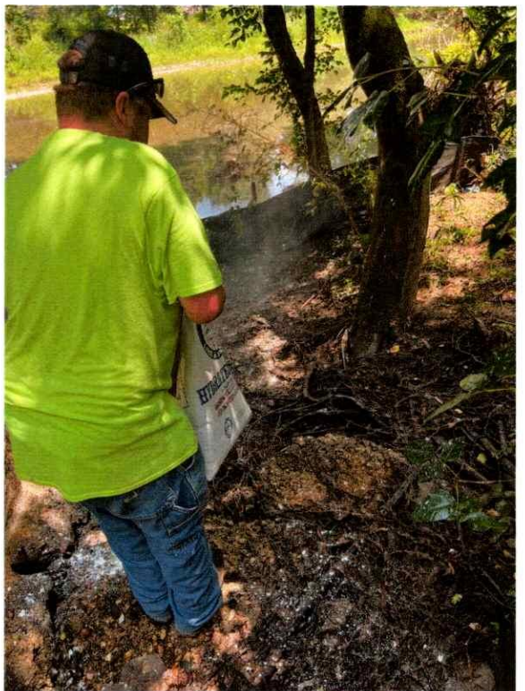
MH 1748 During Cleanup – 7/3/2024
