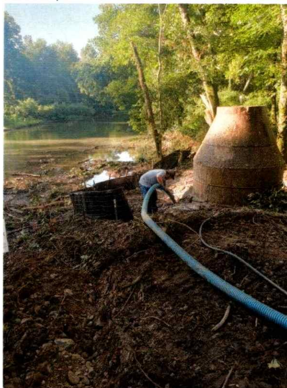
MH 1748 During Cleanup – 7/12/2024
