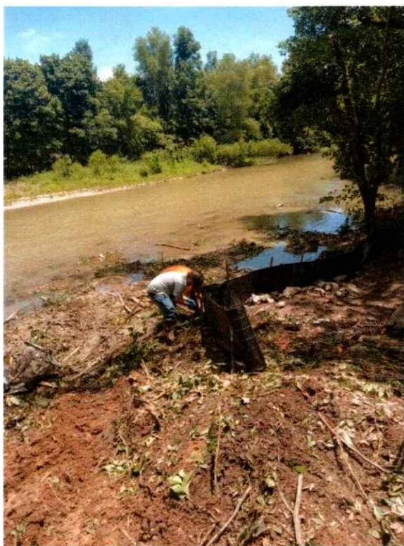
MH 1748 During Cleanup – 7/12/2024
