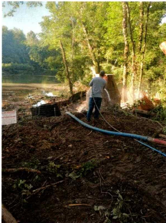
MH 1748 During Cleanup – 7/12/2024
